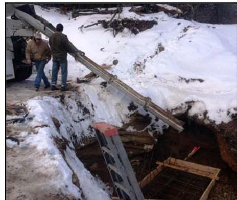
*Right: Footers being poured for the upgrade of the raw water intake.*
