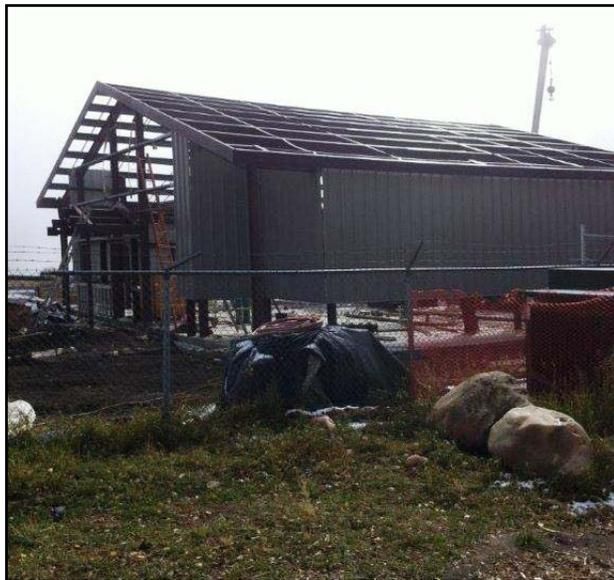
**The walls of the Wastewater Treatment Plant operations building were being installed the first week of October.**
