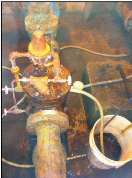
**Corrosion is evident in this photo of the Bridge St. PRV, which is slated for replacement in early October.**
