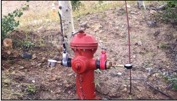
Fire hydrant flushing in Big Springs is in progress. Utilities staff has taken a more comprehensive approach to assessing conditions of hydrants, mapping using GPS, exercising valves, recording flow data, and eventually entering into a data base. Hydrants in Big Springs have been neglected for many years, and many are in need of repairs or replacement. Utilities staff will focus on repairs and upgrades during the month of September. We also have parts ordered
