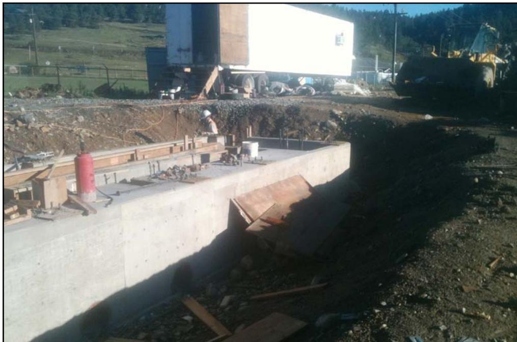
**The head works building, where the intake of raw sewage and initial screening occurs, was constructed in July and August. One feature is mechanized screening of debris, which must be done manually with a rake by Public Works operators at the current lagoons system.**
