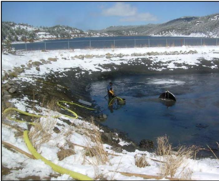
*(Left) A worker from the sludge removal company pumps waste from the north lagoon, in preparation for decommissioning.*
