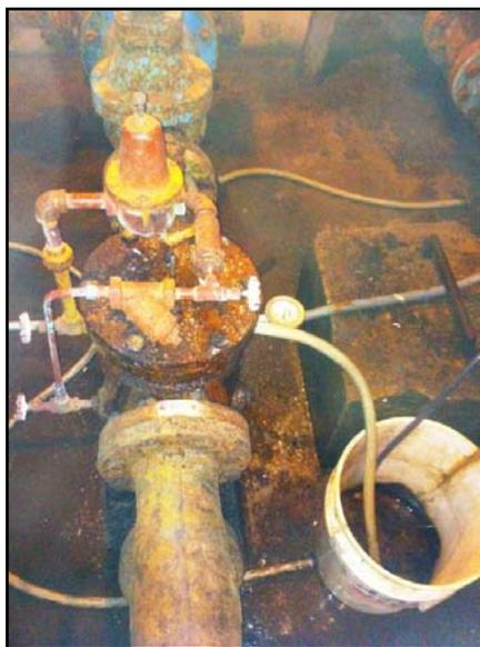
**LEFT: Corrosion is evident in this photo of the Bridge St. PRV, which is slated for replacement.**
