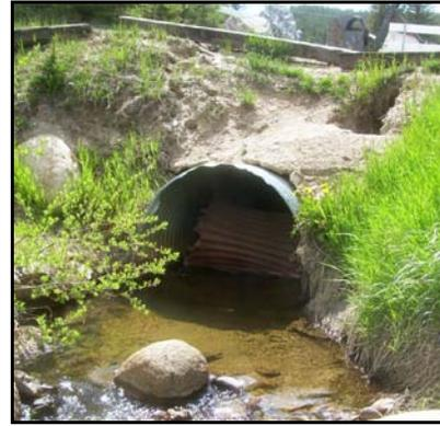
**Right:** In this photo, it is easy to see how the metal culvert had broken down and no longer maintained its structural integrity. As part of the project, the culvert entries were repaired and reinforced with concrete.
