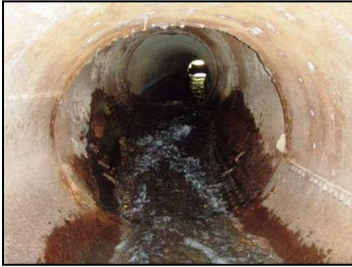
**Left:** This photo of the Bridge St. culvert before repair shows the old metal culvert compacting under the weight above it.
