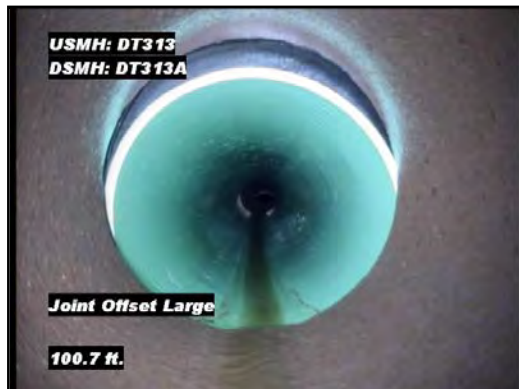
Left: An example of an offset collection pipe, several of which are to be repaired in the project. This pipe is at Conger Street.
