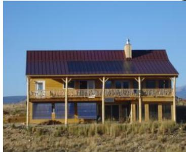
Based on the [movements of the sun](#), passive solar buildings typically have windows (glazing) on the southern facing side\* of the building in order to absorb the [sun's heat energy](#) to warm a building during the winter. In order to stay cool in the summer, passive solar houses rely on a system of [shading](#) (or an overhang) to keep the building cool.
