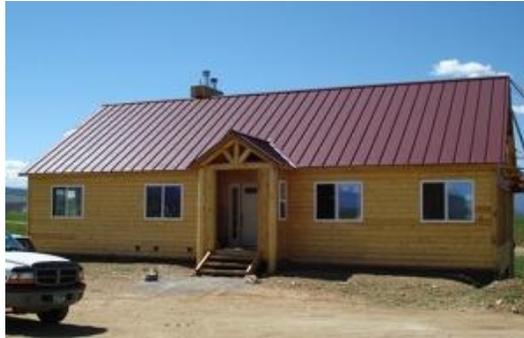
The north facing side of the house has a minimal amount of windows, cutting down on potential heat loss in the winter.
