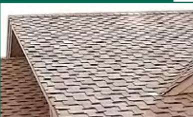
Figure 5-2: Reinforced asphalt shingles
